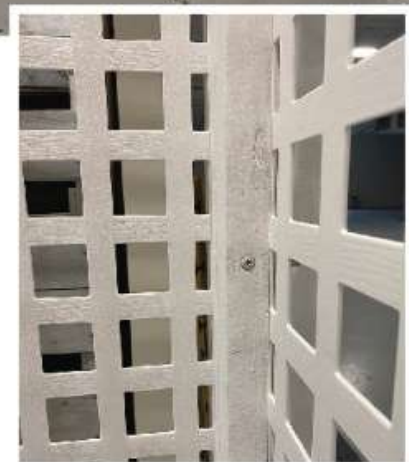
Close up of corner
