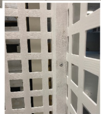
Close up of corner
